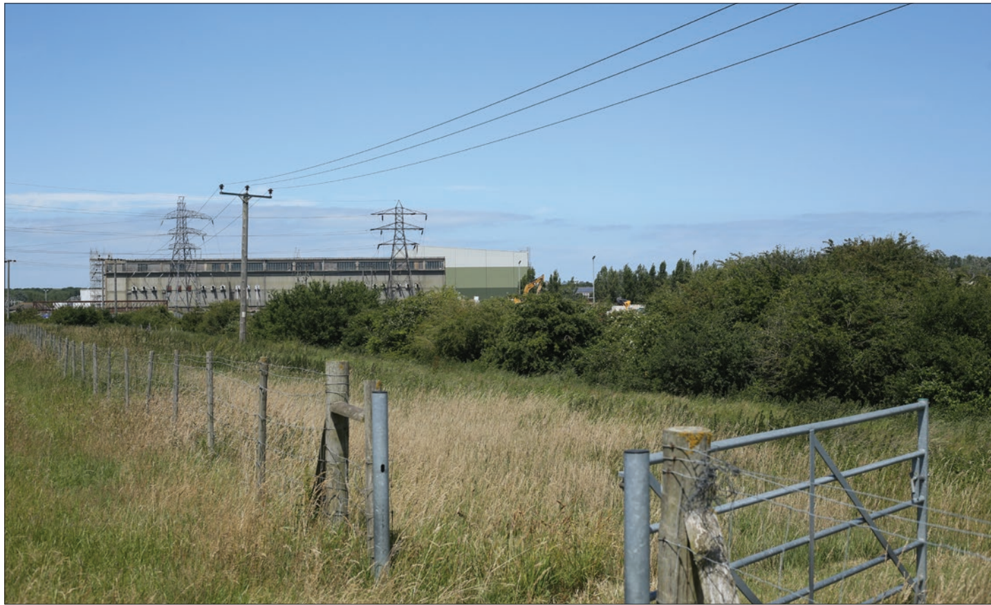
C. View towards existing energy-related infrastructure at south of the Site in Richborough Energy Park seen from Saxon Shore Way (Ash Footpath 42/9)
