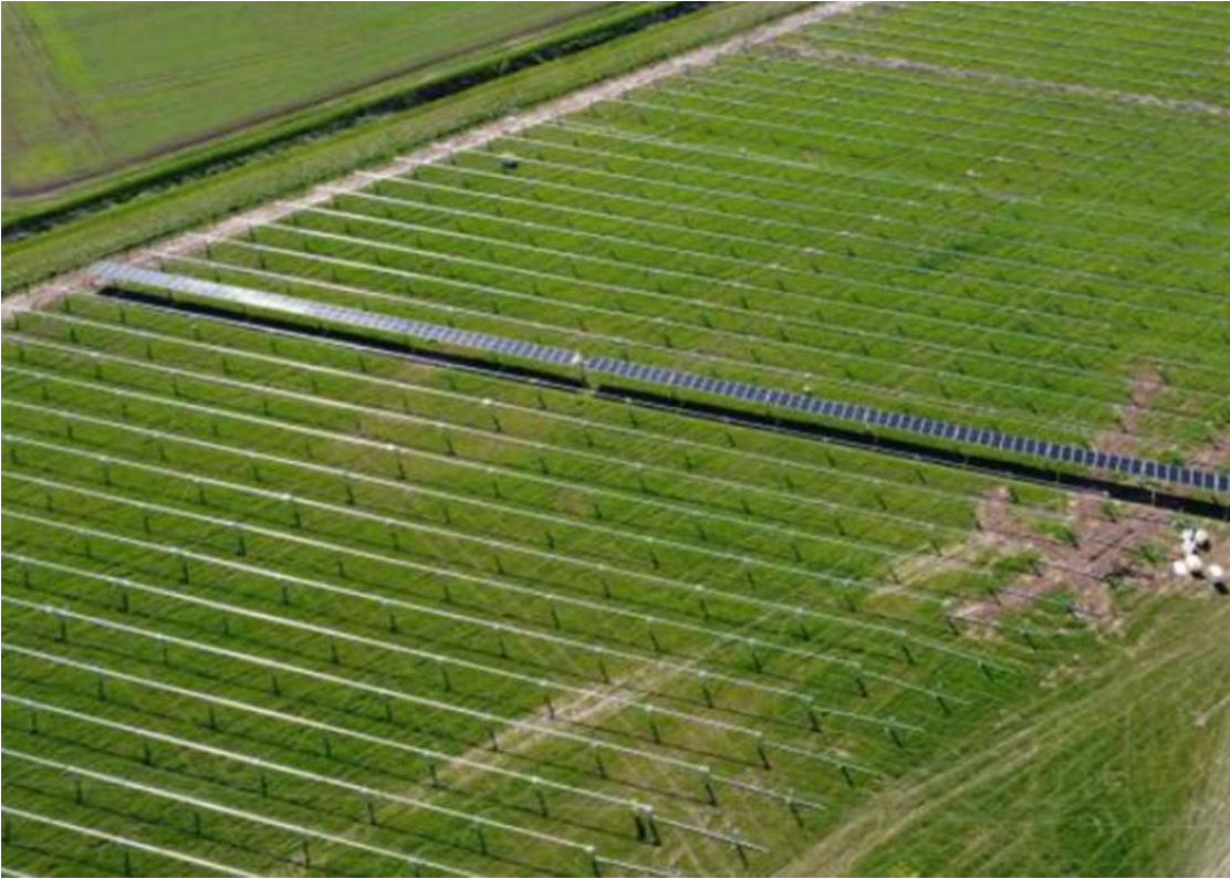
Figure 3 - Solar Panel golden installation completed
