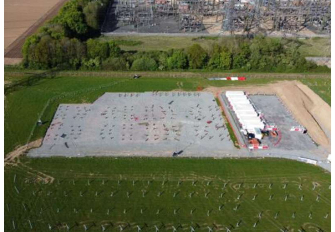
Figure 2 - BESS compound piling completed, structural installation commenced
