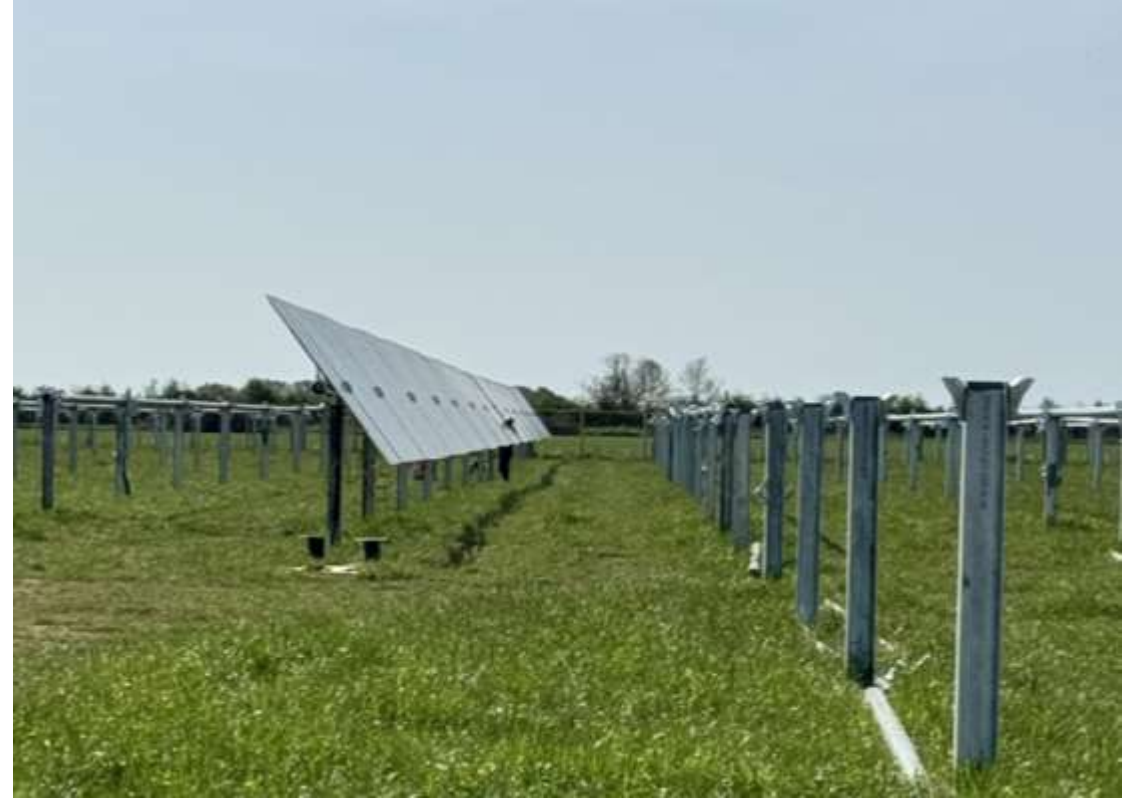
Figure 4 - Solar Panel golden installation completed
