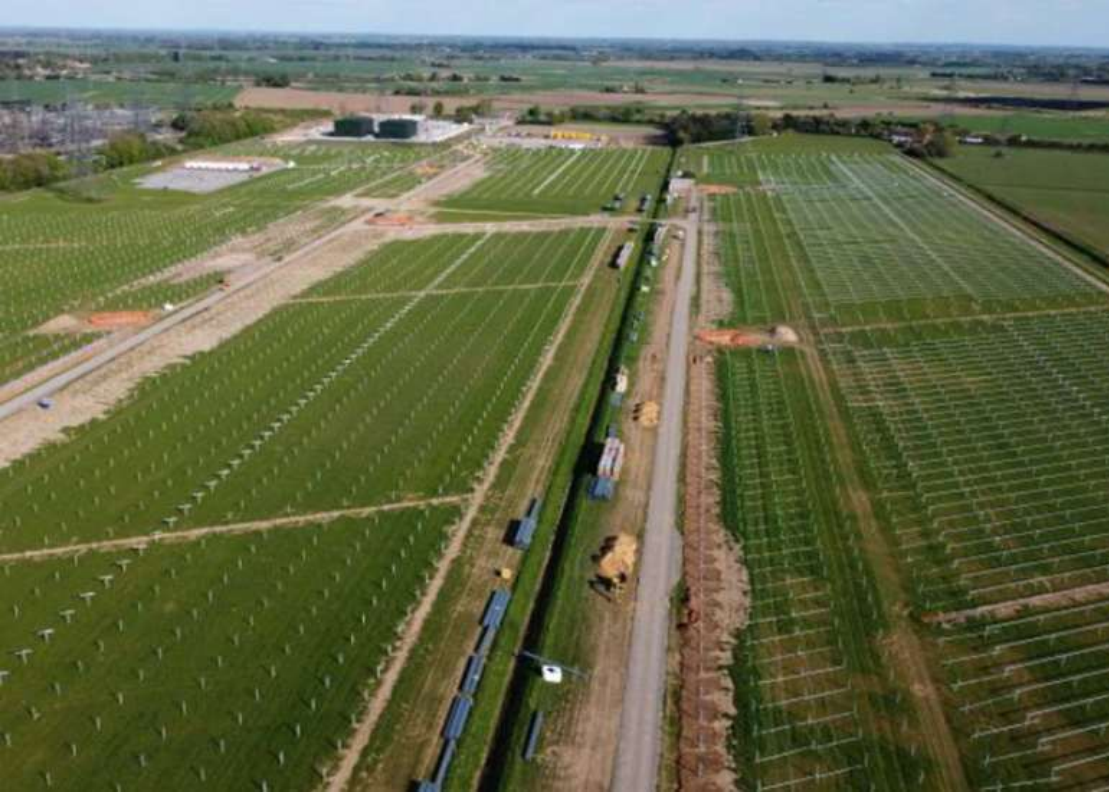
Figure 1 - Solar piling completed, structure installation ongoing
